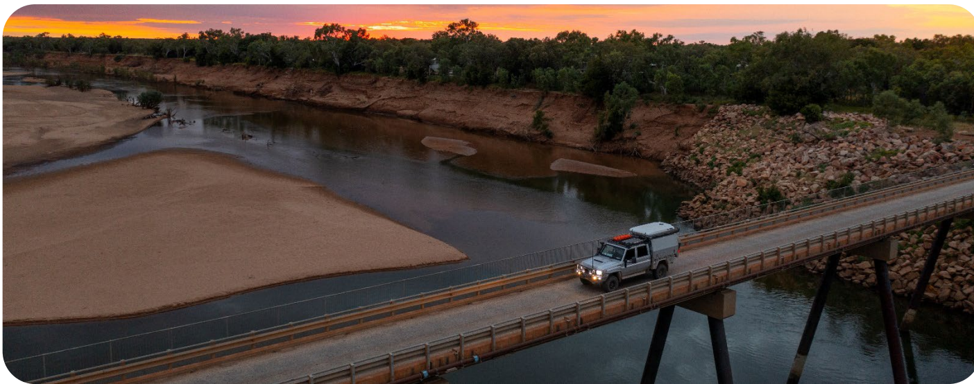
Great Northern Highway (single lane bridge), Fitzroy Crossing. Credit: ANW
